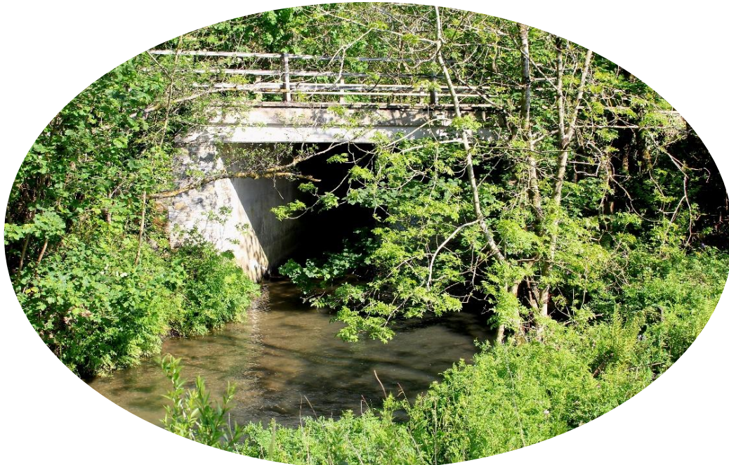
The 'new' A388 road bridge crossing the Lowley Brook at Landue.
