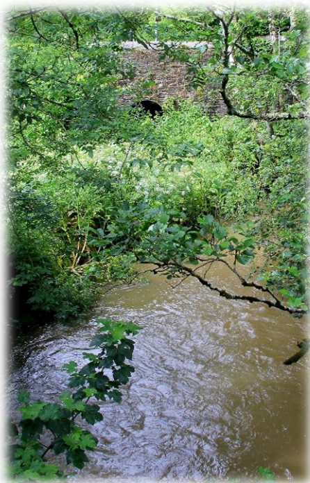
The Lowley Brook at Landue Bridge.
